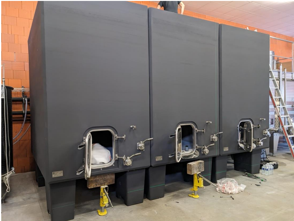
Using a jack for Shimming
