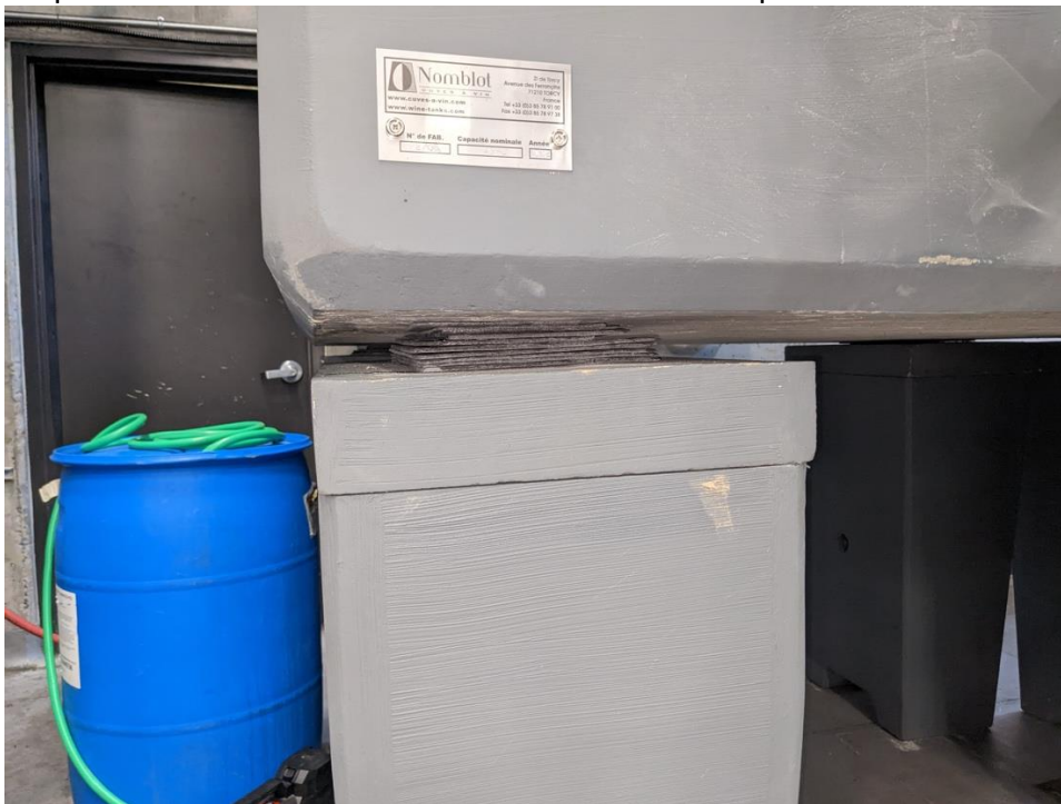
Proper use of Shims between Bottom of Tank and Top of Feet
